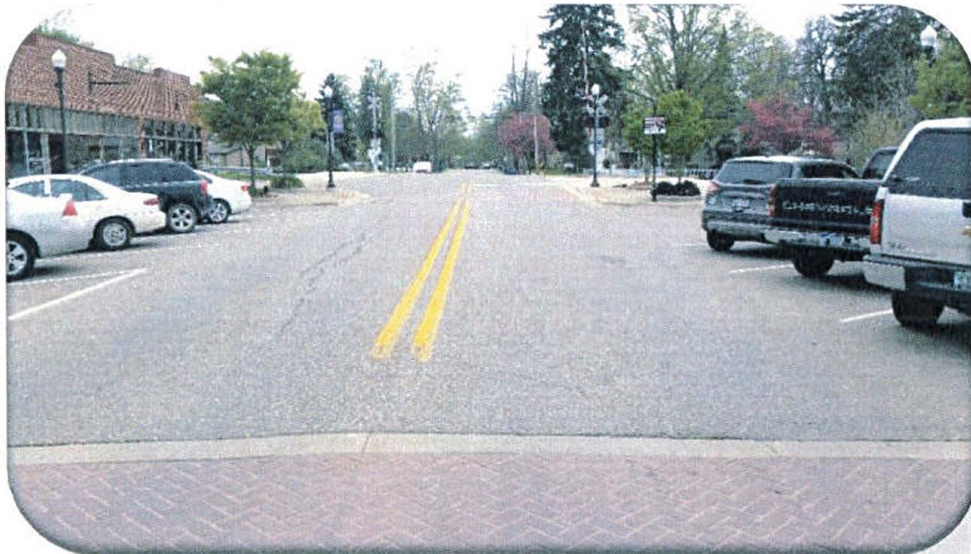
Figure 2: An Example of a Roadway with a Rating of 6
