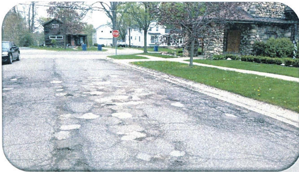
Figure 3: An Example of a Roadway with a Rating of 2
