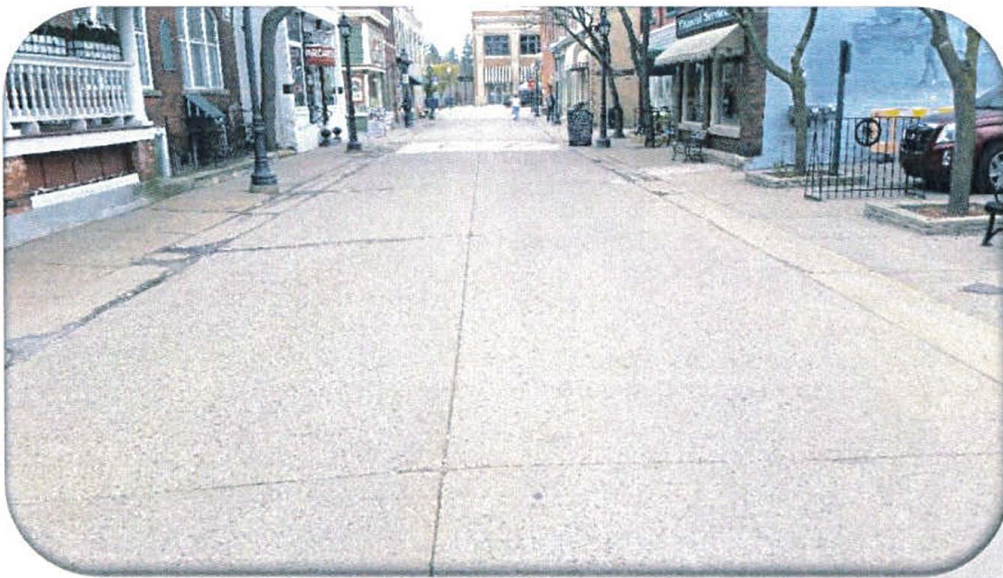
Figure 4: An Example of a Roadway with a Rating of 4
