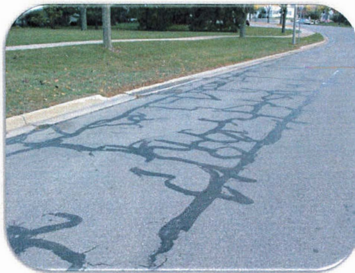
Figure 5: An Example of a Roadway Treated with Crack Sealing
