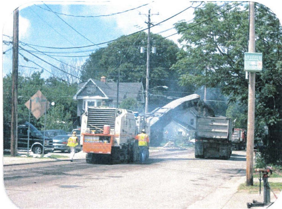
Figure 6: An Example of a Roadway Being Treated with a Mill and Resurface
