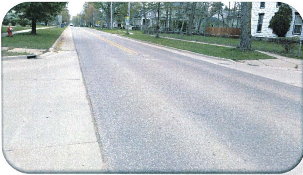
Figure 1: An Example of a Street with a Rating of 7
